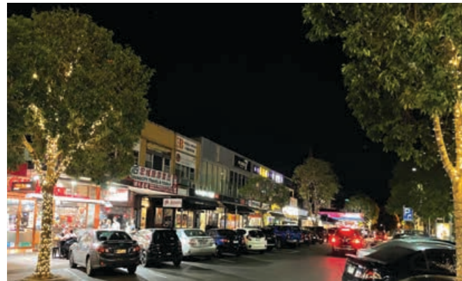
Feature lighting, Glen Waverley
