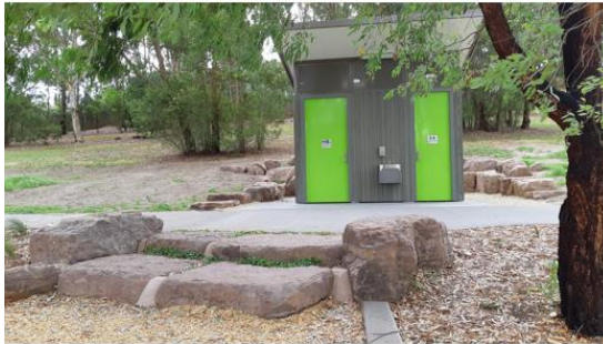
Public Toilet (Jenkins Park)
