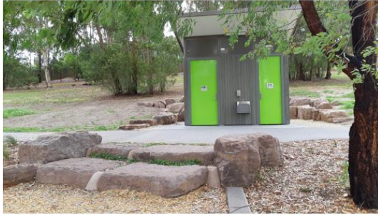
Public Toilet (Jenkins Park)
