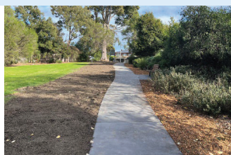
Tolsoy Footpath Construction
