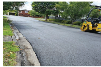
Saxonwood Drive Resealing Works
