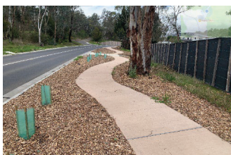
Jumping Creek Road
