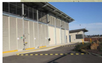
Example of spill capture bund within roadway
