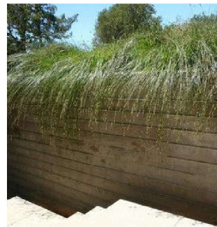
Potential retaining wall options: a) and b) in situ concrete with timber form work
