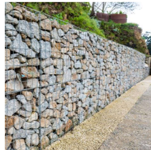
c) Gabion wall
