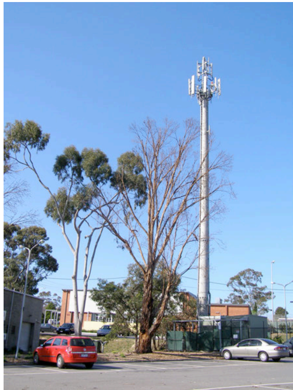
Photo 12: Telecommunications Tower at rear of existing Scout Hall
