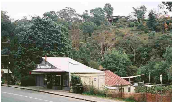
View to the north of Yarra Street showing a shop which is low in form with a pitched roof allowing views to the treed valley and down to the river. The building steps down the slope rather than cutting into the embankment.
