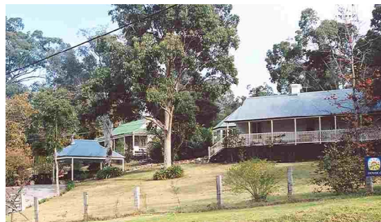
Significant residences at the east end of the precinct
