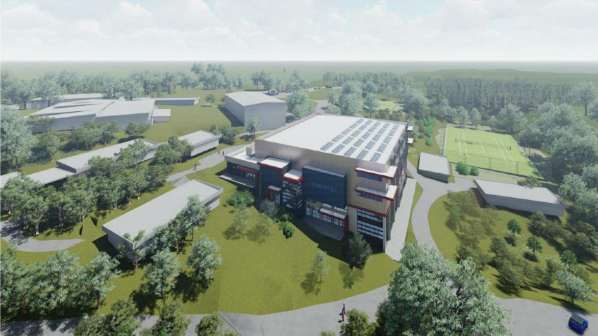
EAST ELEVATION AERIAL
