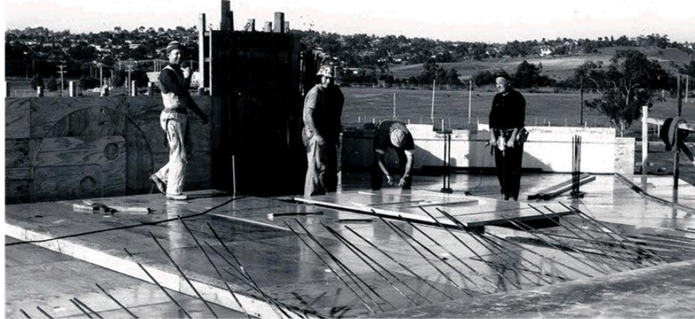
Image 5: Original Veneto Club Building in construction
