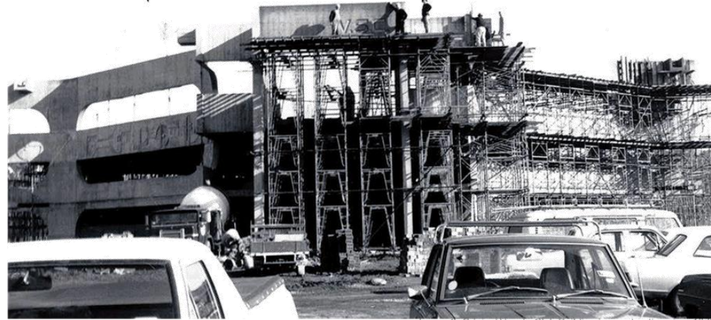
Image 3: Original Veneto Club Building in construction circa 1972
