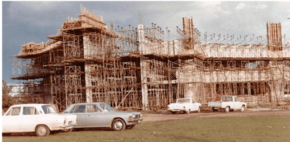
Image 6: Original Veneto Club Building in construction
