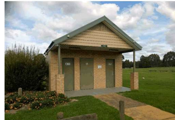
B. Standalone facility with unisex self-contained toilets – manually maintained.
