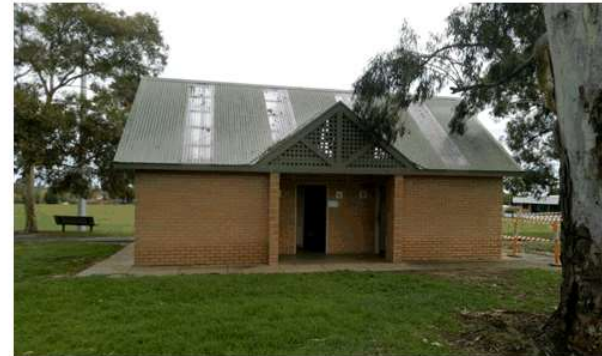
A. Older style standalone facility with gender segregated toilets.
