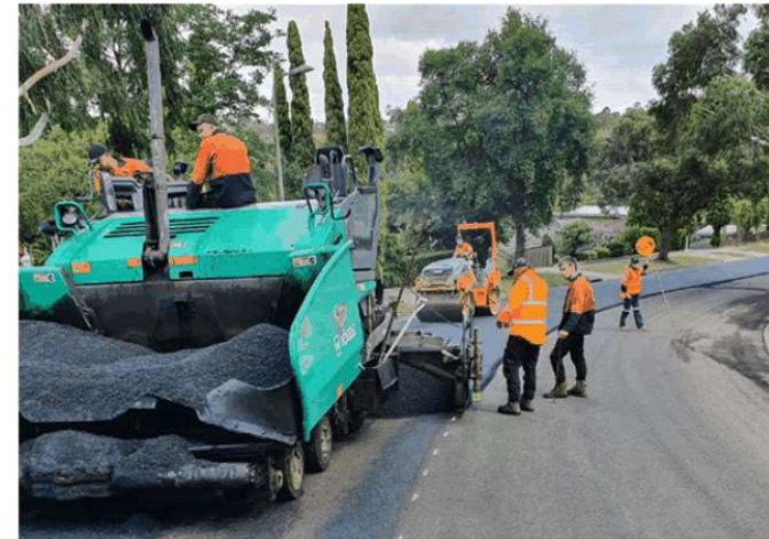
Resurfacing Works - Clontarf Crescent, Templestowe
