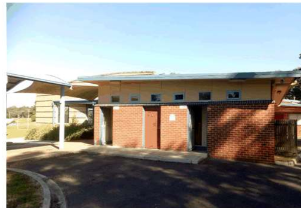
D. Independently accessed toilet facilities, under same roof as a pavilion or other building. Mix of unisex and gendered toilets.
