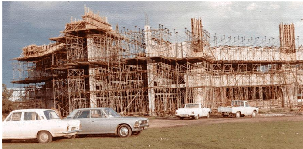
Image 6: Original Veneto Club Building in construction
