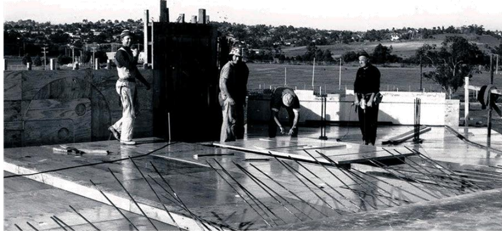
Image 5: Original Veneto Club Building in construction
