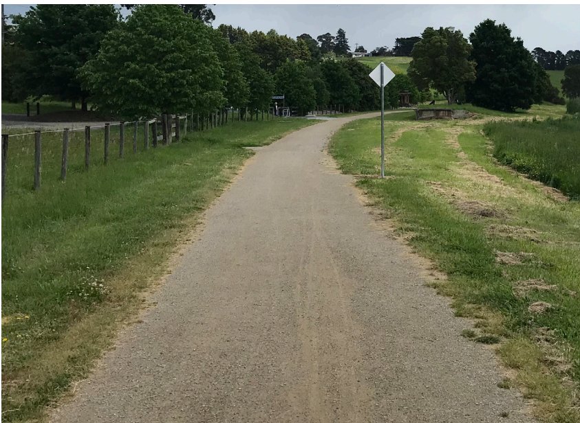
FIGURE 8.1: Regional trail construction material examples. Top: Concrete trail construction (Heathmont Belgrave Trail) Middle: Asphalt surface with concrete strip edging (Anniversary Trail) Bottom: Gravel (Warburton Rail Trail)
