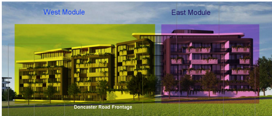
Figure 7: Southern Elevation identifying East and West Modules (view from Doncaster Road)
