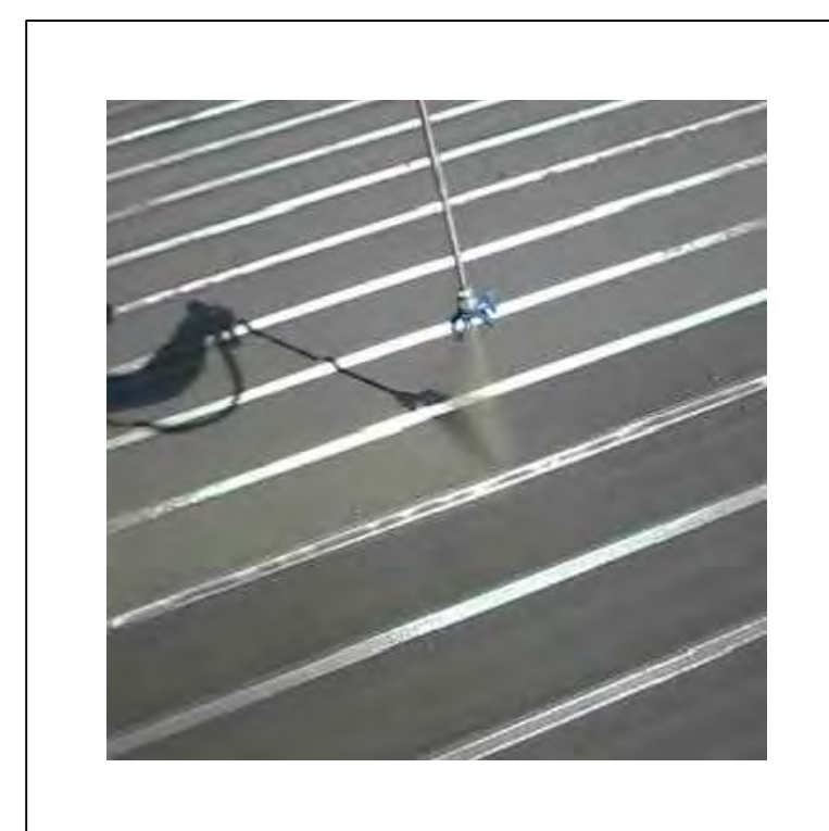
MATERIAL 15: SELECTED METAL ROOFING
