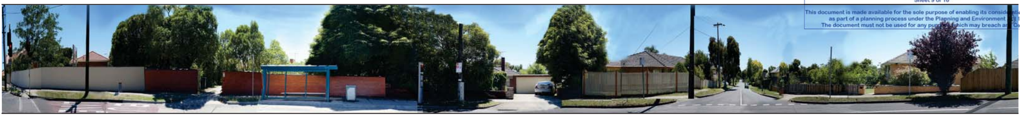
01 Existing Streetscape Photo Doncaster Road
