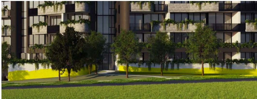
Figure 18: Southern Elevation of Main Entrance (including 3.0m high southern retaining walls adjacent)
