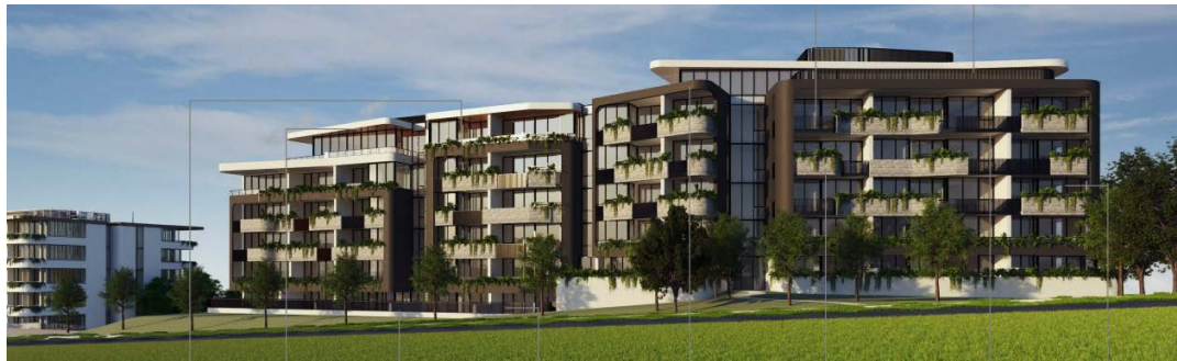
Figure 5 – Southern Perspective of building from Doncaster Road (recessing of upper levels)
