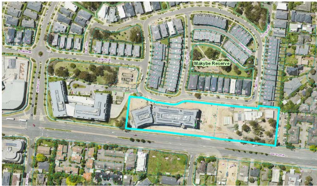
Figure 2: Aerial view of the subject site within the southern portion of the Tullamore estate (December 2020)
