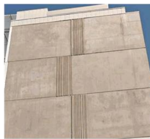
Example of use of P2- Precast Medium Grey oxide on a facade of a building
