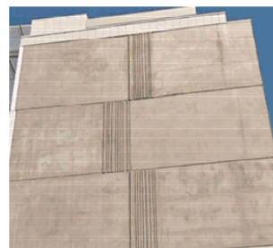
Example of use of P2- Precast Medium Grey oxide on a facade of a building
